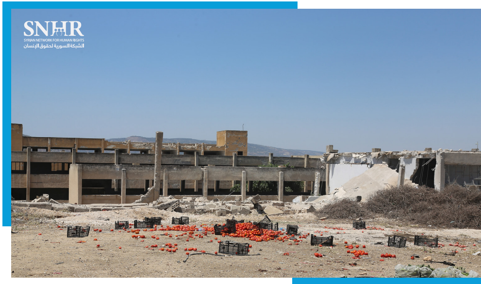
Damage to the vegetables market in eastern Jisr al-Shoghour city in rural Idlib following a Russian airstrike that resulted in casualties - June 25, 2023 | Photo credit: Abdullah Saed ©SNHR
